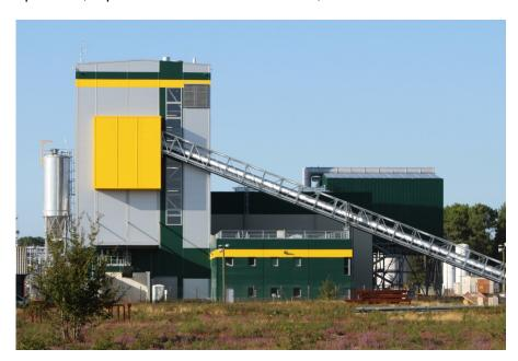
The Biomass Energy Solutions VSG plant at the DRT site in Vielle-Saint-Girons is now in operation. The tested performances are well within the guaranteed values. The boiler efficiency is approximately 93%.
