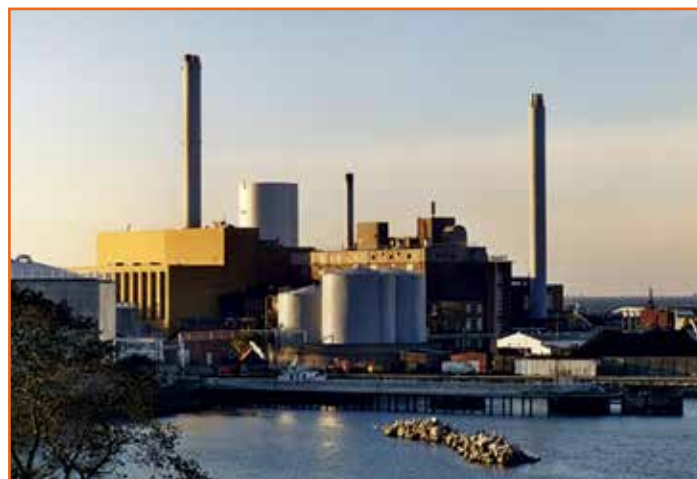
The Østkraft plant on Bornholm island
